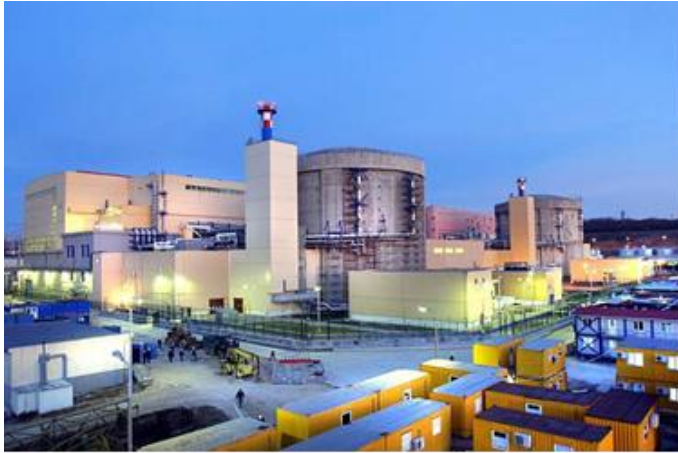
Fig. 1.2a Cernavoda NPP Units 1 and 2
