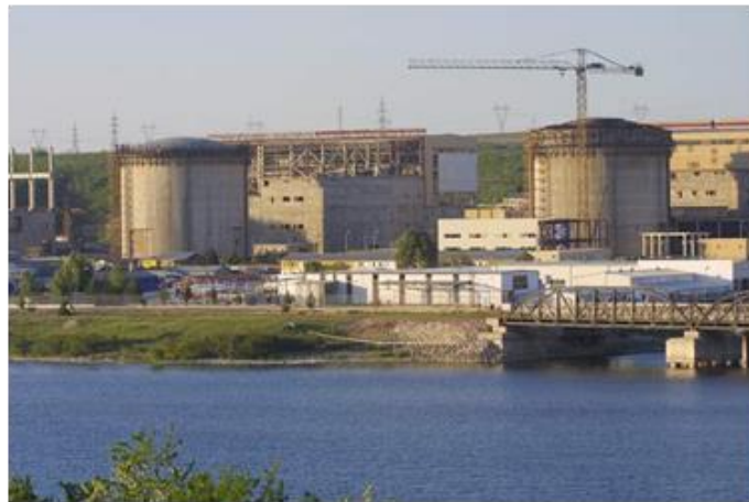
Fig. 1.2b Cernavoda NPP Units 3 and 4
