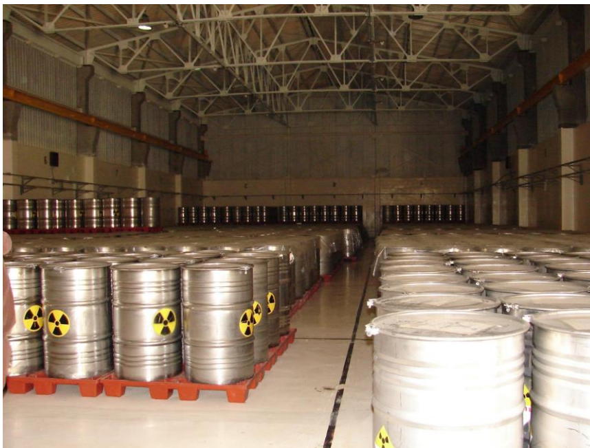
Figure B6: DIDR - The structure no. 1 – warehouse inside
