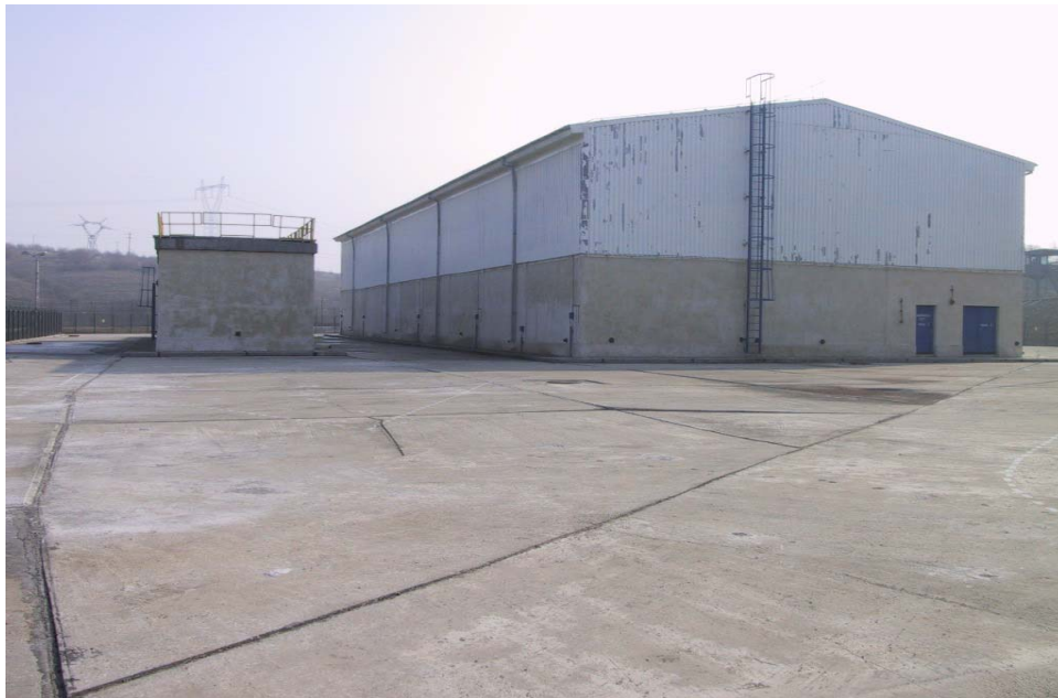
Figure D3.1-1: DIDR – outside view
