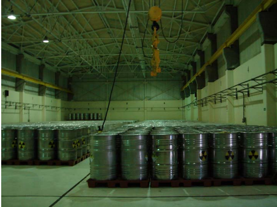
Figure D3.1-2: DIDR - The structure no. 1 – warehouse inside view
