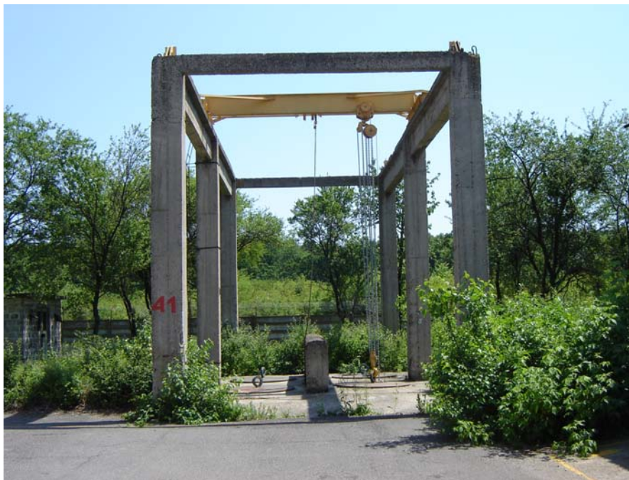
Figure D3.4-1: Spent Filters Storage Facility (DFU)
