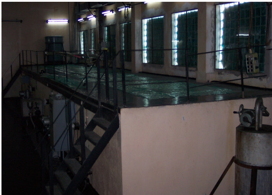
Figure D1.3-1. Spent fuel storage ponds at the VVR - S Reactor of IFIN-HH
