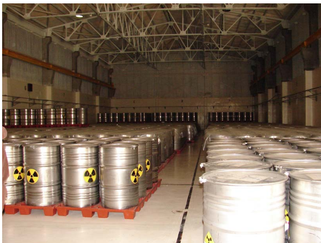
Figure B8: DIDR - The structure no. 1 – warehouse inside view
