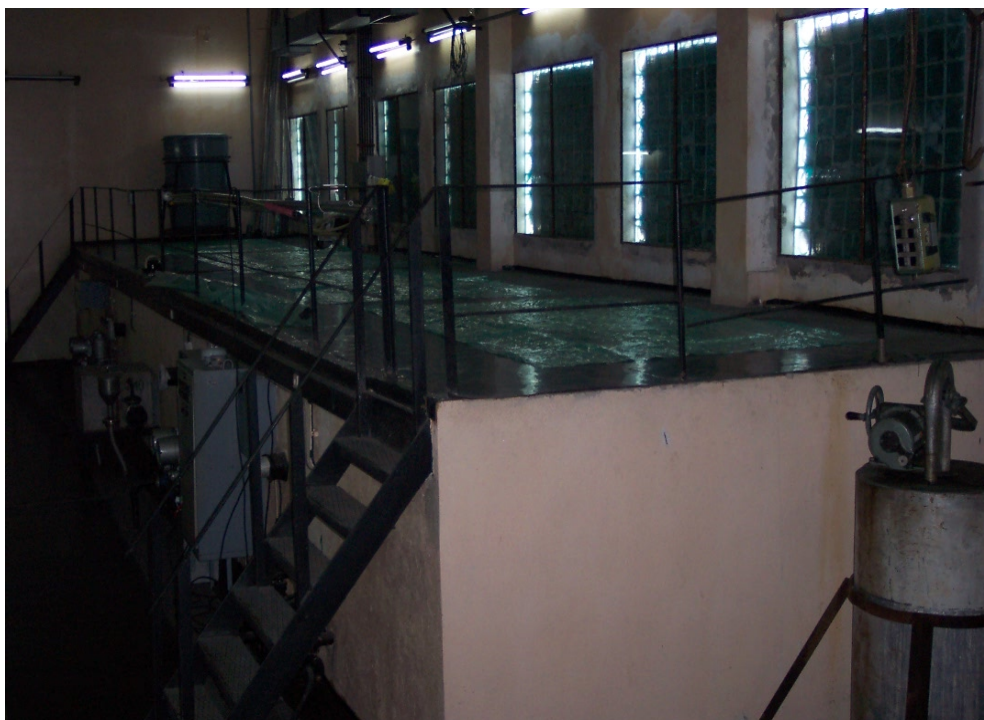
Figure B6. Spent fuel storage ponds at the VVR - S Reactor of IFIN-HH
