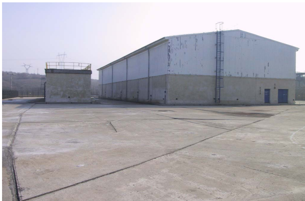
Figure B7: DIDR – outside view
